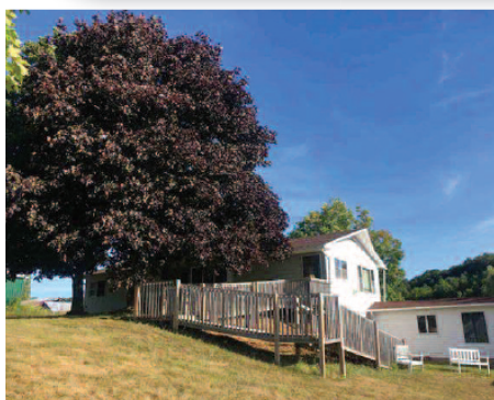
02106 S ADVANCE ROAD • EAST JORDAN
